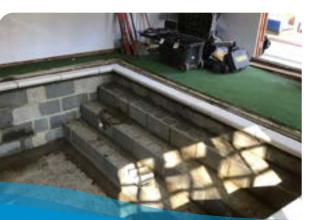
Nestled in the heart of North London, this aging indoor swimming pool was in dire need of a comprehensive refurbishment. The existing steel liner pool had fallen into disrepair, plaqued by leaks and corrosion that rendered it unsafe and unsightly. Our team was commissioned to breathe new life into it, tasked with constructing a new reinforced concrete pool within the existing excavation.
